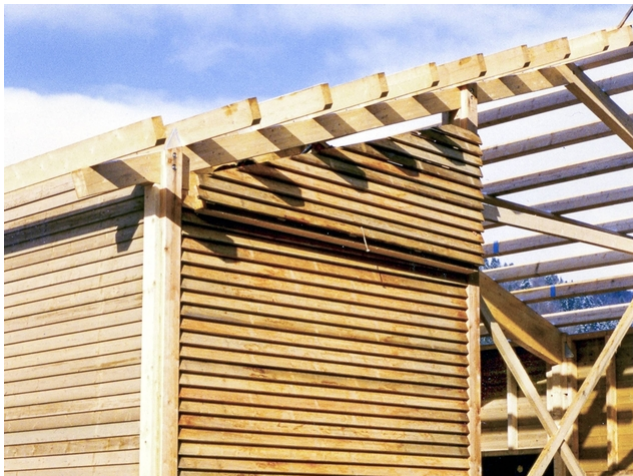
Assembly of the wall elements
