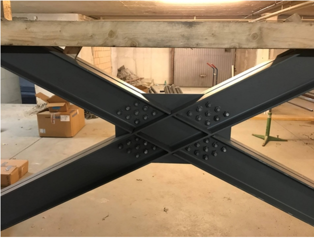
Steel cross for earthquake reinforcement
