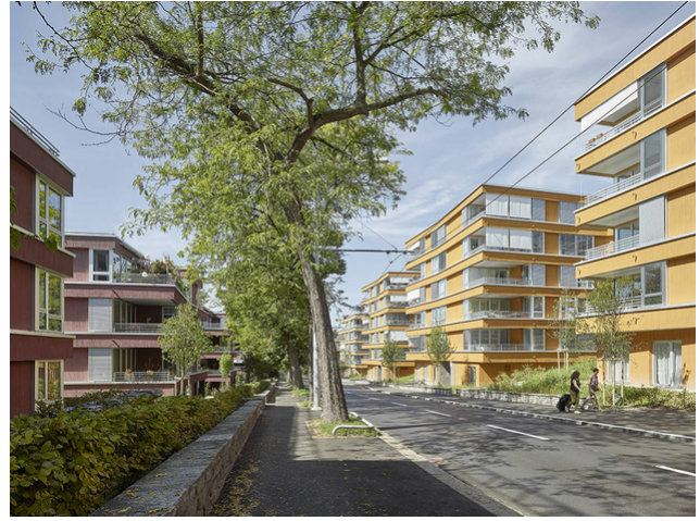
Road side 1st and 2nd stage
