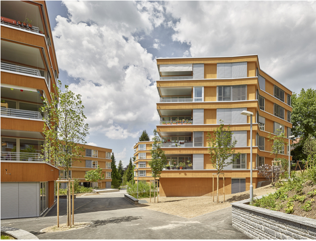
Exterior view 2nd stage
