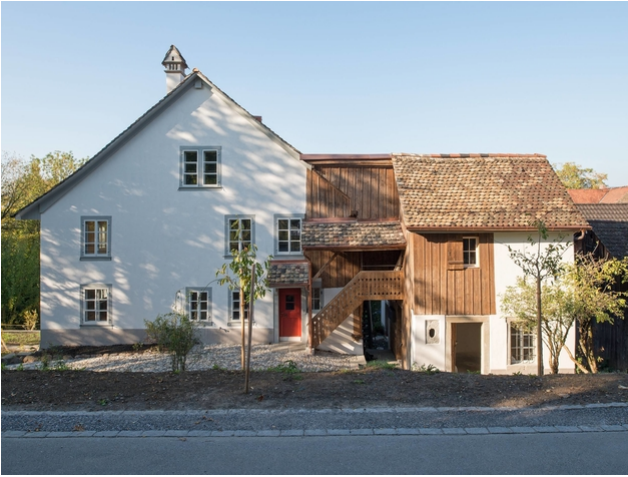
View from the street side
