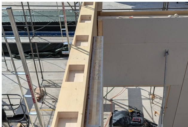
Milled pockets for accommodating the shear cams of the Vierendeel truss
