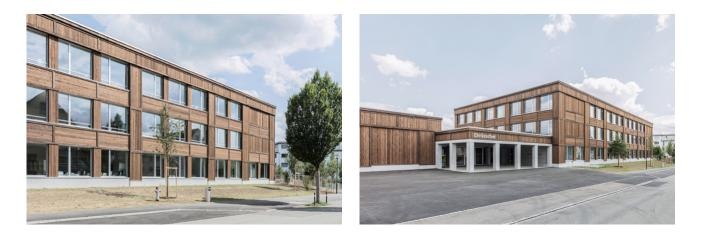
On the initiative of Timbatec, the new school complex in Bassersdorf ended up with even more wood than planned. Originally, only the walls of the gymnasium were to be made of wood, while the roof was to be made of concrete. Timbatec suggested that the roof should also be made of wood in order to save costs.
