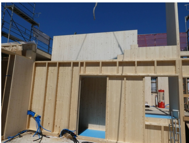
Assembly of wooden construction elements
