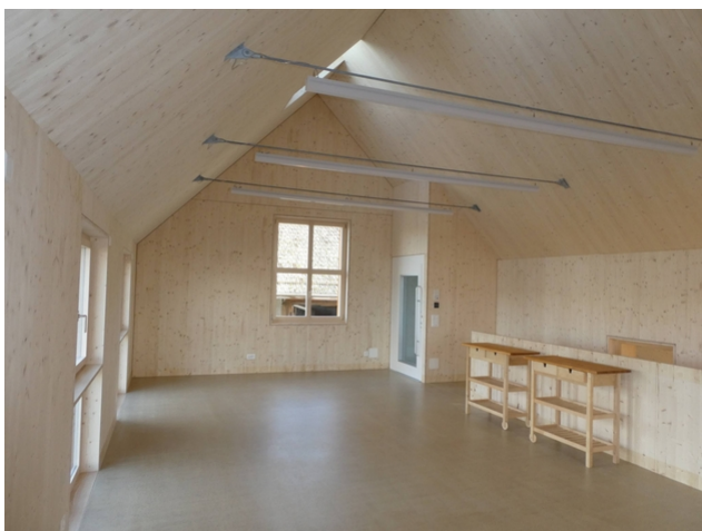
Tie rod for absorbing the static forces
