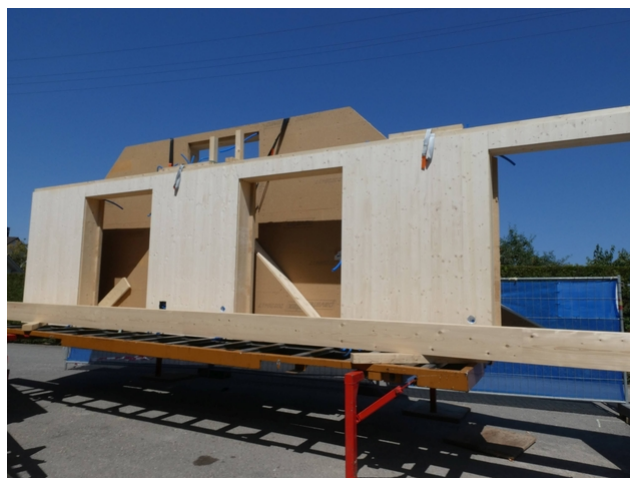
Delivery of the wooden construction elements
