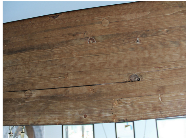
Failure of glulam beams
