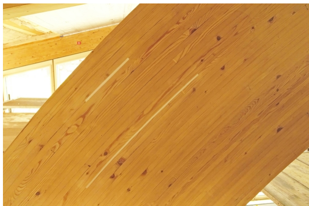
Detailed view of a rehabilitated adhesive joint
