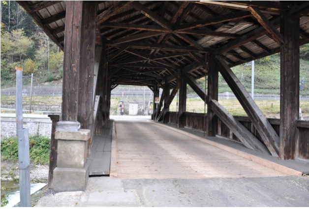
New roadway with oak boards surrounded by air
