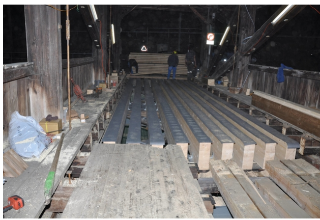
Assembly new side member at night
