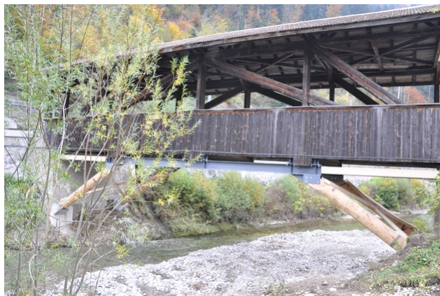
View of the bridge after renovation
