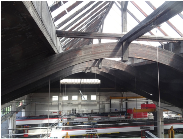
Arch truss with drawstrings
