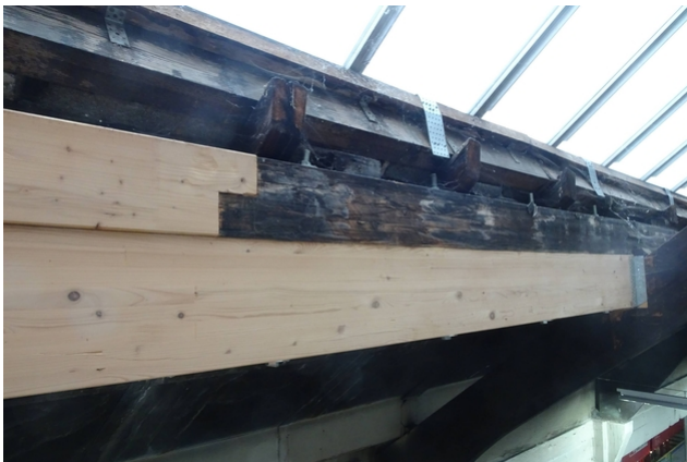
Replacement rafter purlins
