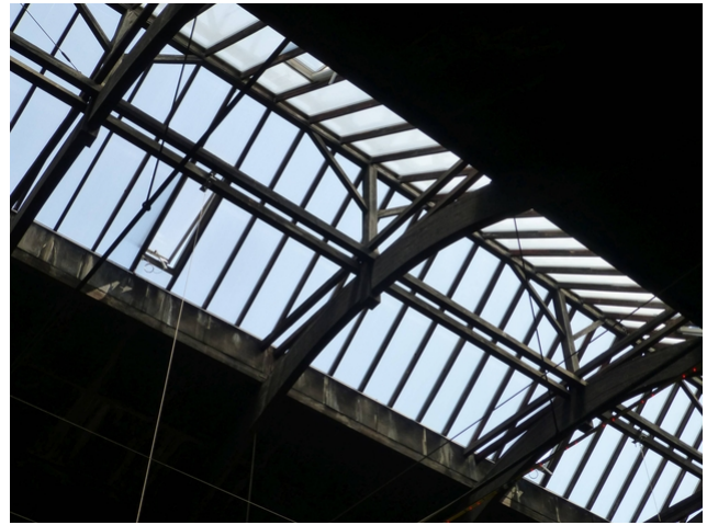
Interior view roof
