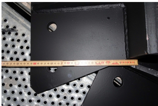
Reinforcement of the beams with metal parts
