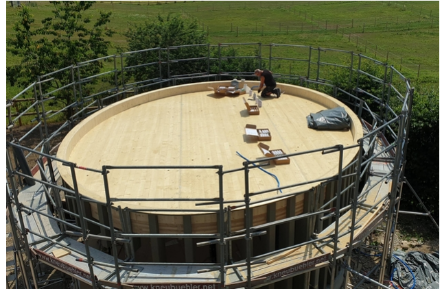
Grouting the TS3 joint
