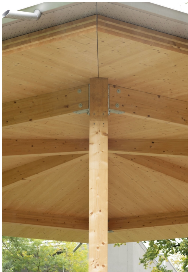
View of corner posts including beam connections
