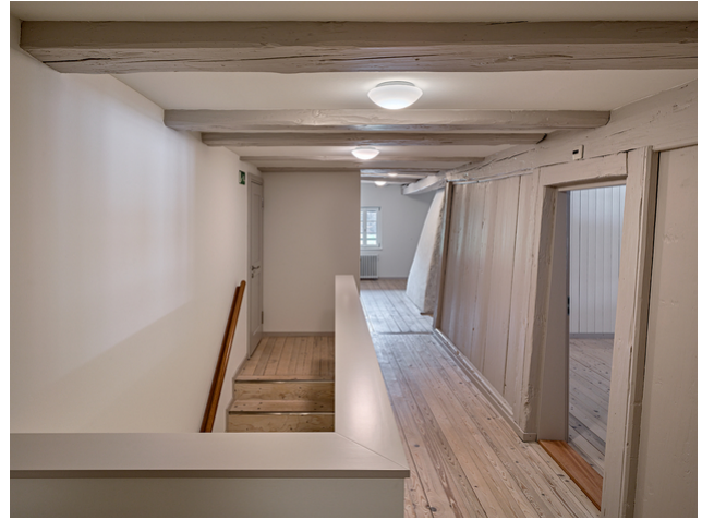
New fire protection cladding was inserted between the existing beams
