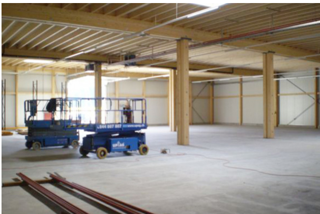
Interior view carcass
