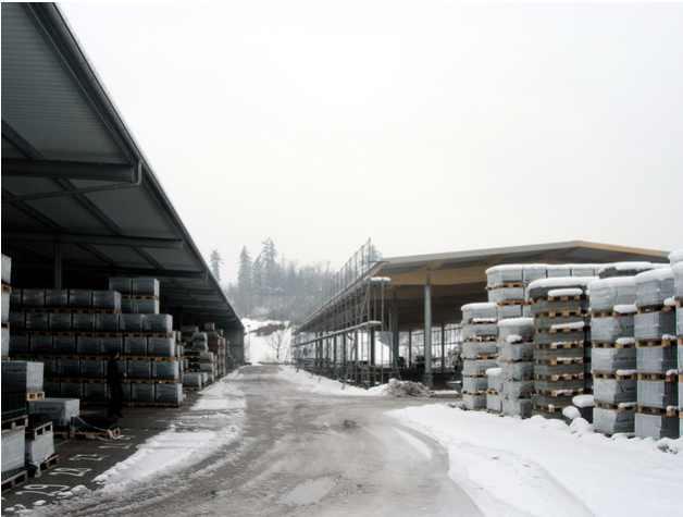
Old and new roofing
