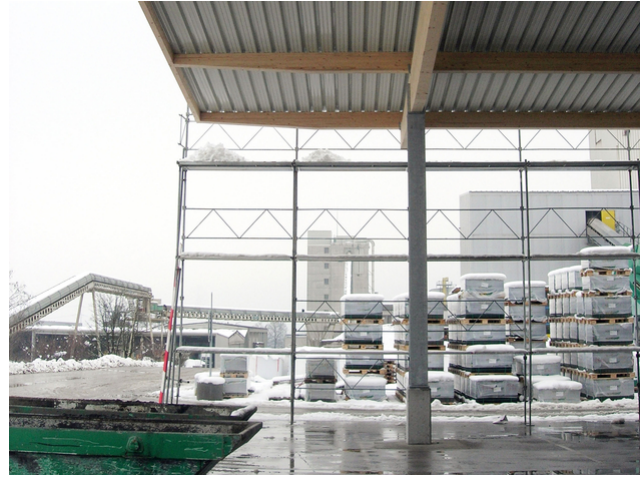
Steel column and wooden truss
