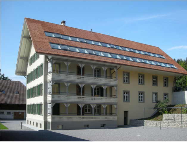
Mill building renovated
