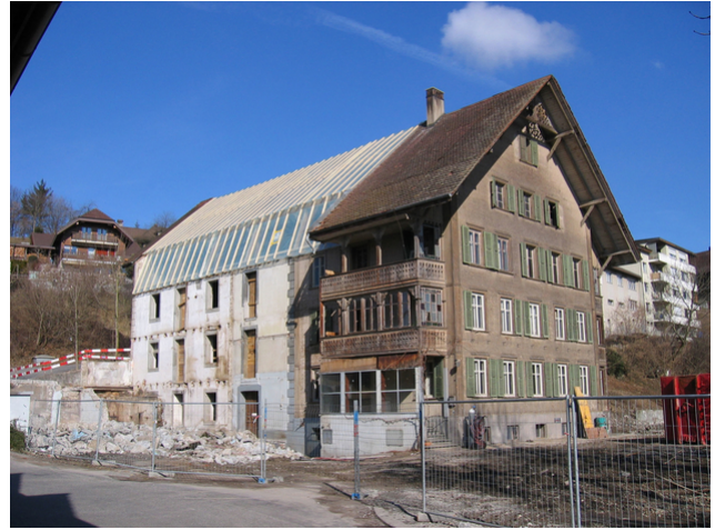
Mill before renovation
