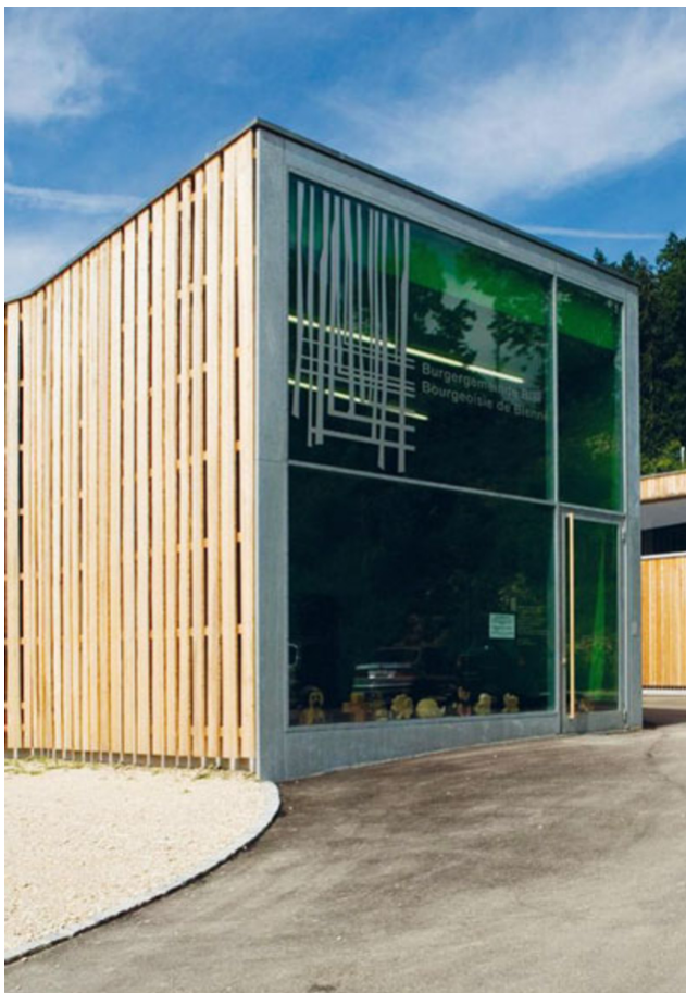
Detail view entrance
