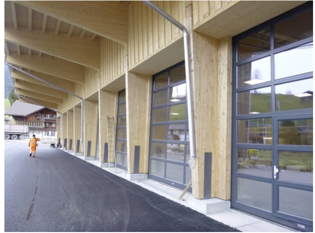
The building is almost entirely made of local wood and bears the Swiss wood origin mark (HSH)
