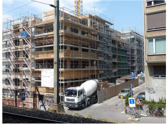
Shell erected
