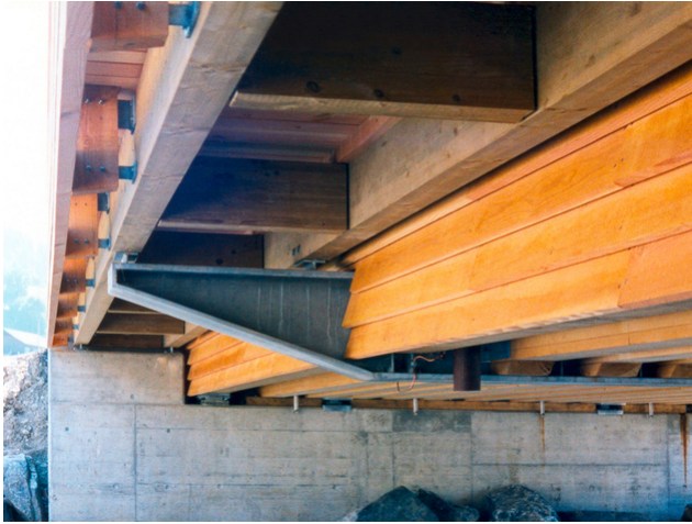
Built-in steel cross member
