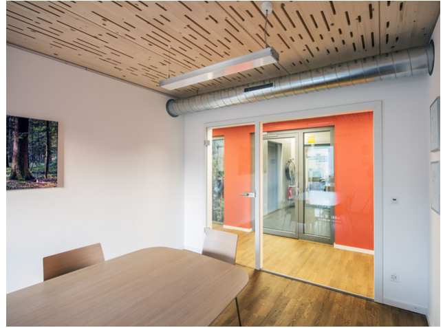
Feature: Lignum ceiling elements with acoustic holes
