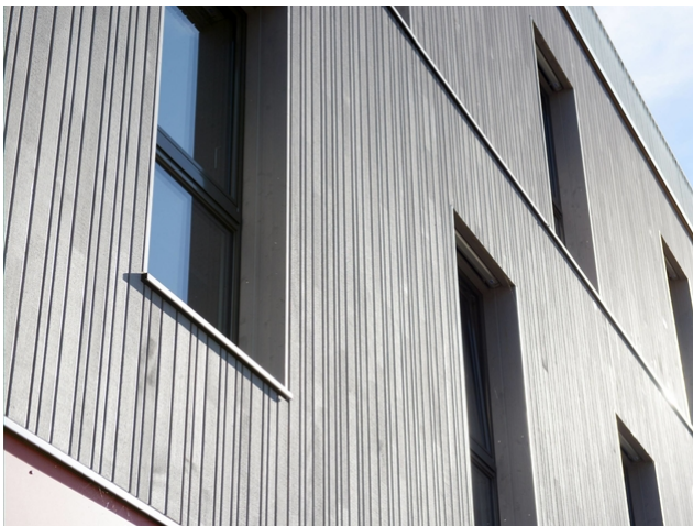
Versatile: Facade with materials from the OLWO range
