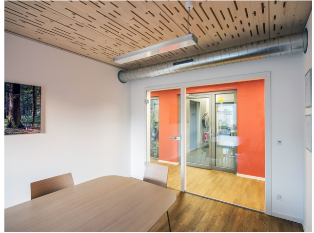
Feature: Lignum ceiling elements with acoustic holes
