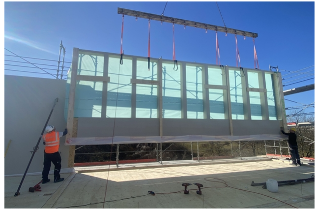
Erection of prefabricated wall elements
