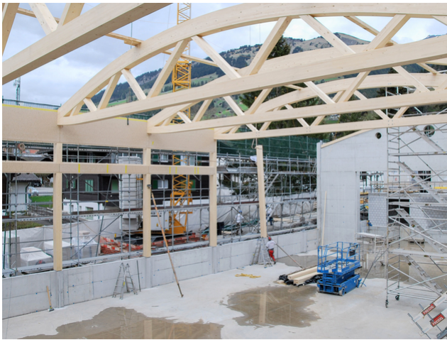
More supporting structure height due to the slightly upward curved bottom chord of the trusses
