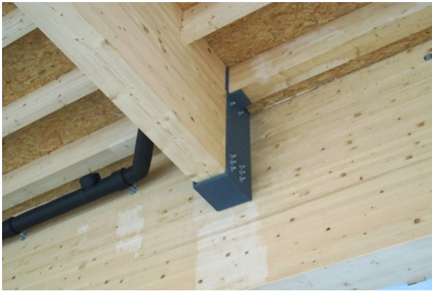
Roof support detail
