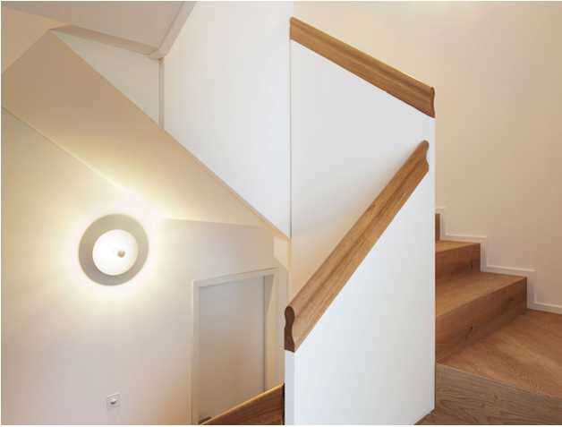
Both the flights of stairs and the stair landing were made of wooden structure
