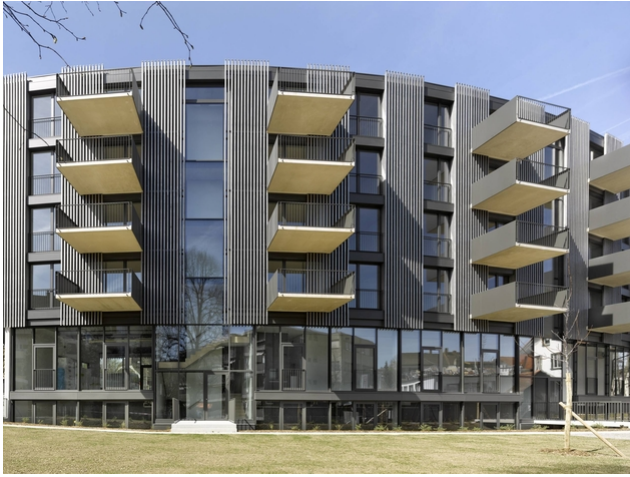
Facade view with balconies
