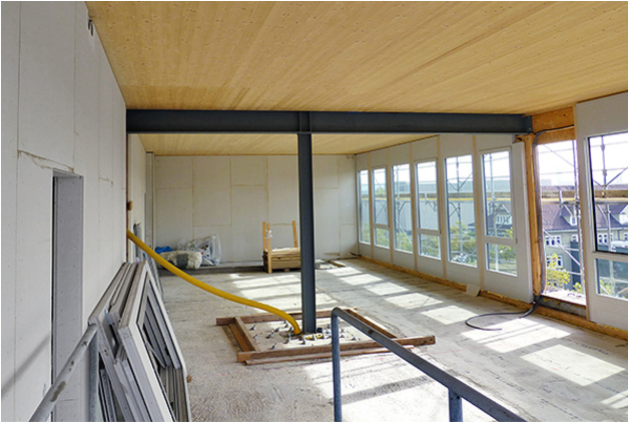
Primary steel structure
