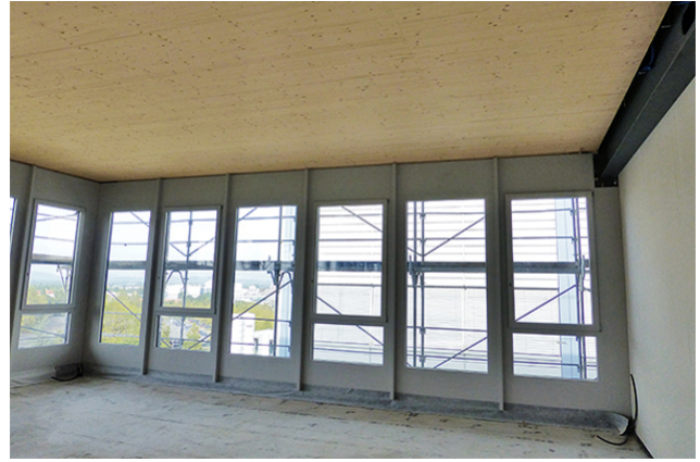
Wooden ceiling with 9m span
