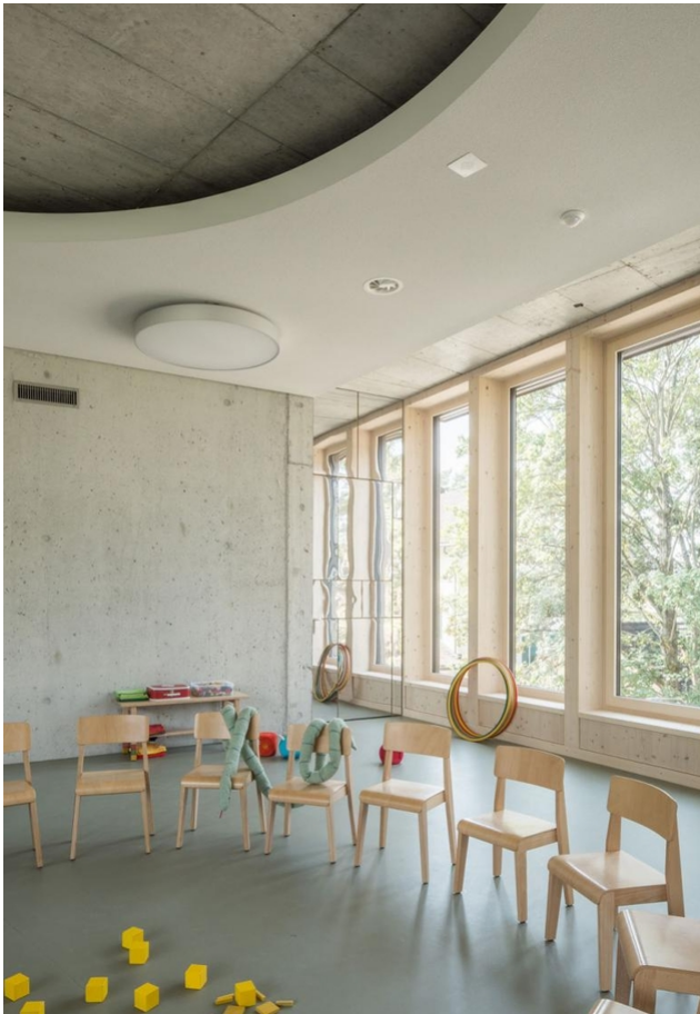
Interior view: facade in wood. Above lies the concrete ceiling
