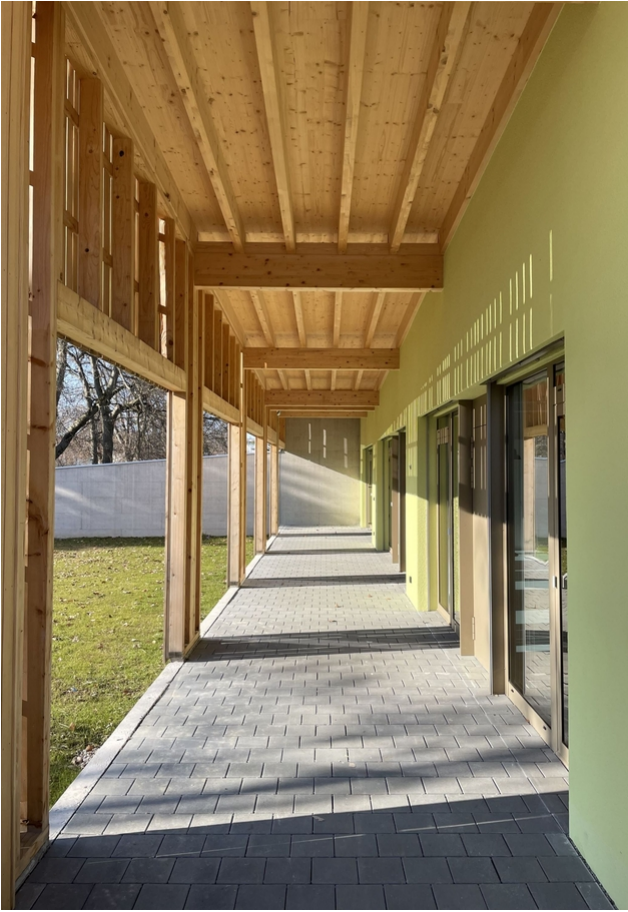
The portico with the visible joists
