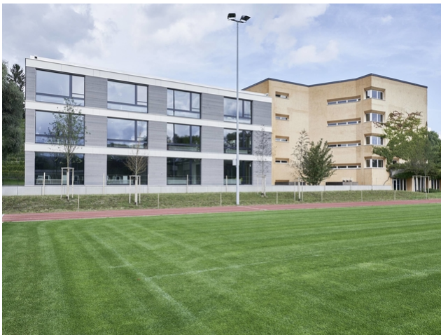
The newly designed surroundings of the school facility in Oberengstringen
