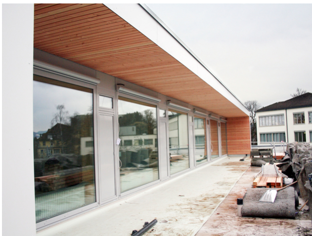
Facade view extension north side
