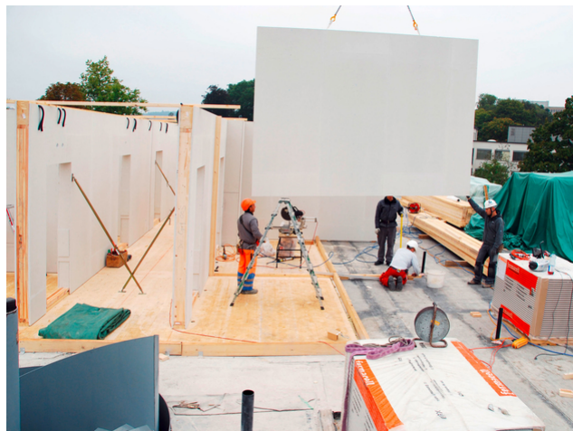
Relocation partition walls addition
