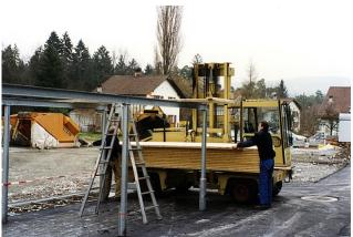
The architects envisioned a wooden slab laid over two steel girders - with a span of 4.50 meters. The plate was to be no more than about 4 cm thick and covered with greenery. This was not feasible, because with a construction less than 110 mm thick, the deflection would have been too great. But such a thickness would have been neither aesthetically nor economically satisfactory.
