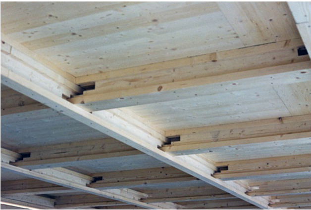
Finished beam grate
