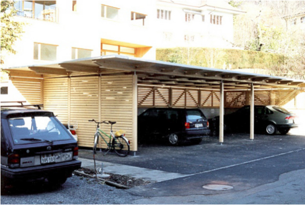
Finished car shelter
