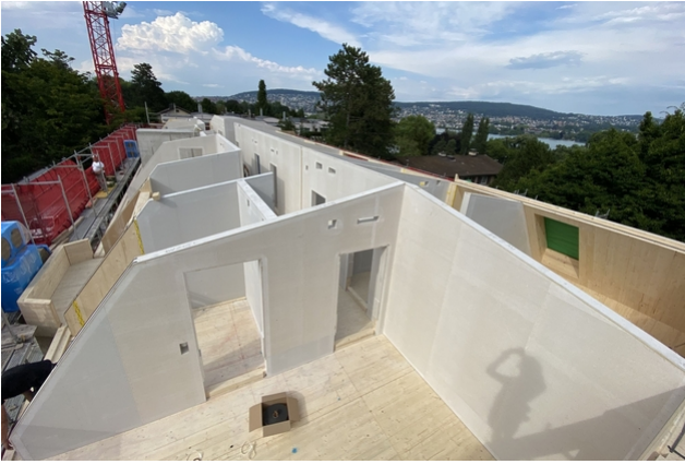
View directly into the element construction elevation
