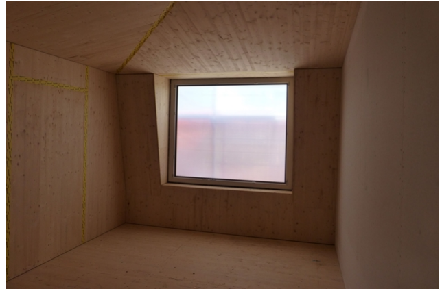
Interior view during the construction phase
