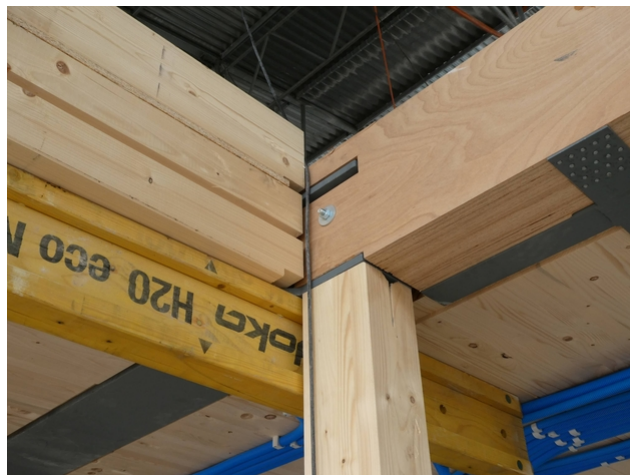
Beams made of beech wood
