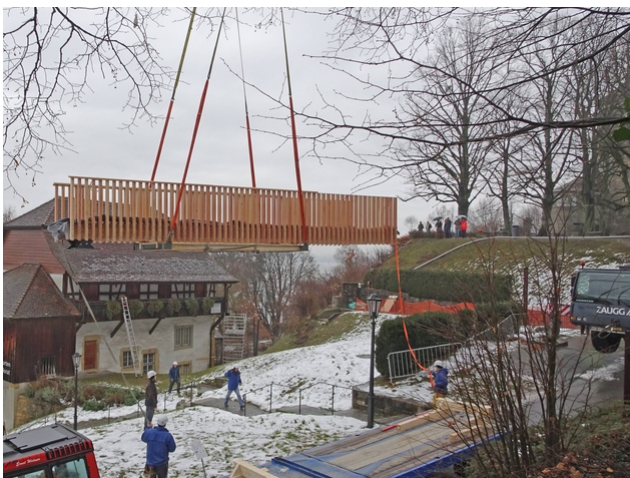
A crane lifted the 10.5 meter long bridge into place
