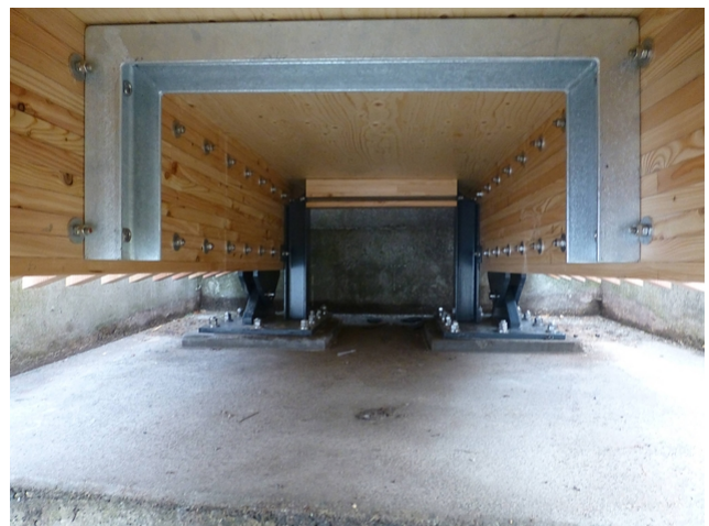
The new bridge was clamped into the existing abutment niche
